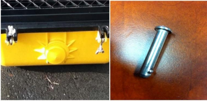
Picture 3 - Door shall have stainless steel eyebolts with wing nuts, and hinge pins that are removable without using tools.
