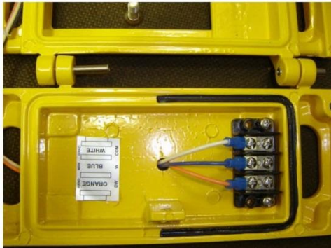
Picture 4 – clamshell with 3 position terminal
